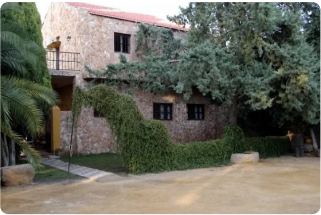
WEB The side elevation and the gravel court in front of it.
